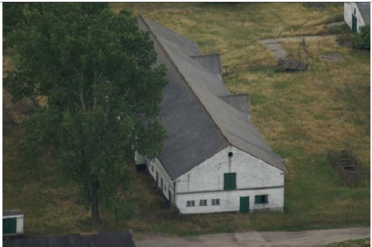
Large abandoned Farm building housing a very significant hydroponic cannabis crop
